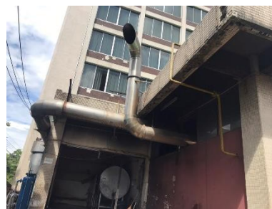
Figure 2. Flue gas of boiler is released to surrounding
