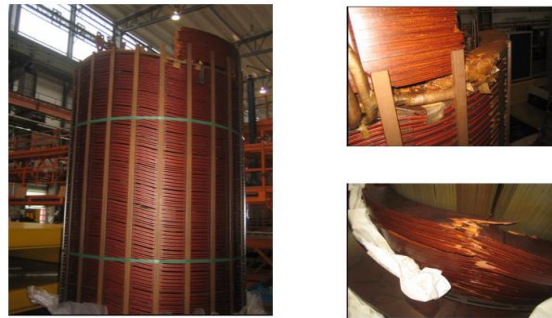
Case 6 Internal inspection
