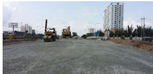
Figure 8. Pavement was recovered after treatment
