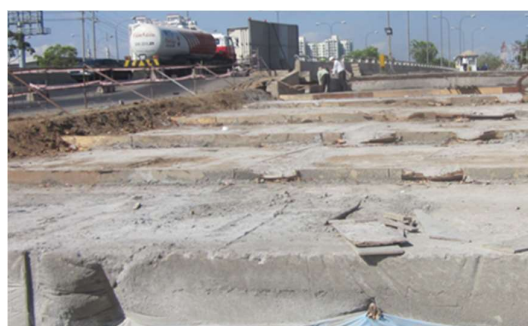
Figure 5 – Body of embankment using lightweight concrete – front view
