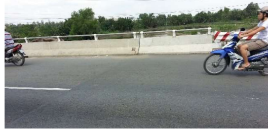
Figure 7. Approach was still smooth after 7 months in traffic
