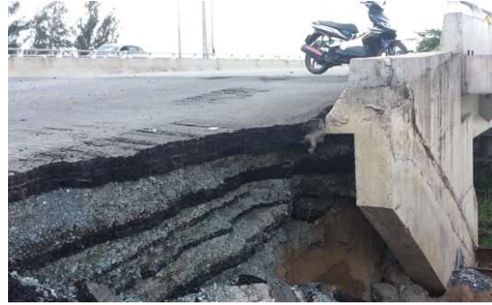
Figure 1. Approach was levelled by crushed aggregate and asphalt concrete many times
