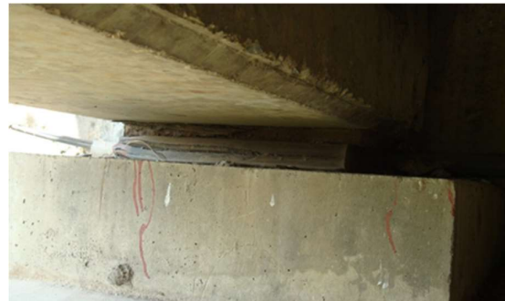
Figure 3. Bearings appeared oblique displacement, steel pith was posed without rubber covering layer
