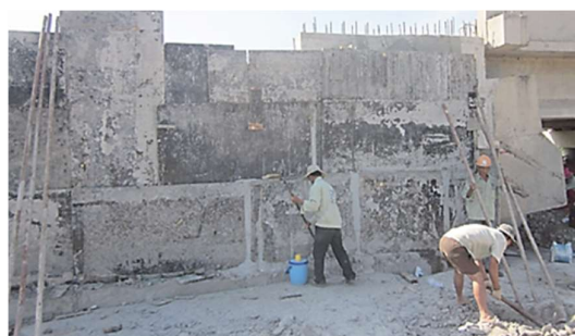
Figure 6 – Body of embankment using lightweight concrete – side view (under construction)
